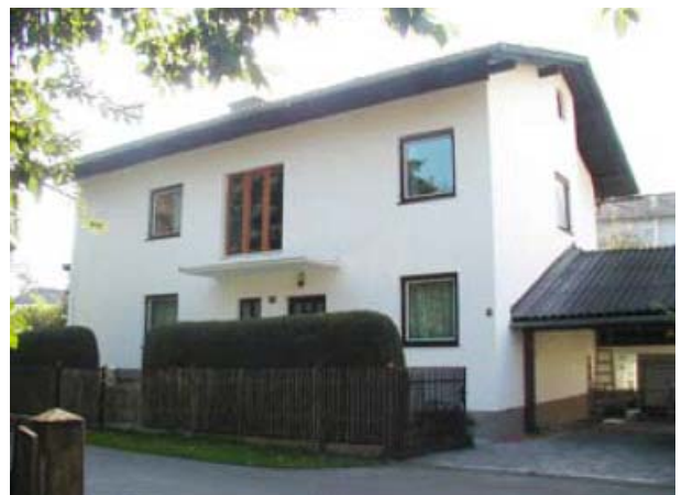
Shielding paint has been covered with sealer and top coat.
